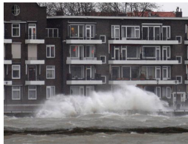
Along the River Meuse, buildings are not much higher than the high water level. As water levels continue to rise, the chance of flooding increases. PHOTO PETER HILZ
